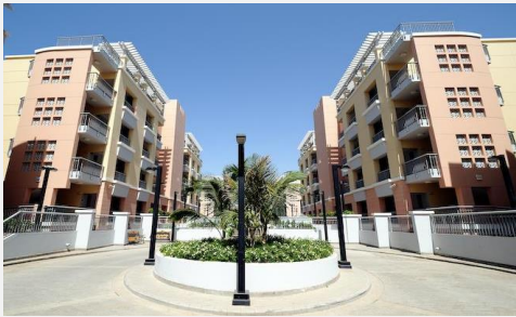
Sukoon Hospital Building
